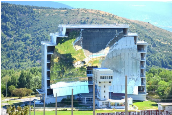
Solar Furnace (Man-Made Solar Concentration) The Odeillo Solar Furnace focuses sunlight to produce temperatures of 3,500°C for scientific research.
