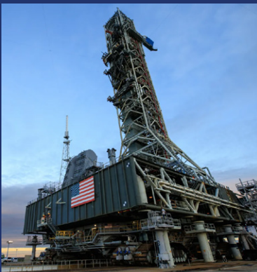
Launch pad ground support equipment
