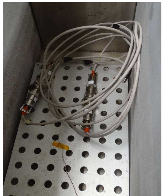
Connectors inside refrigerator
