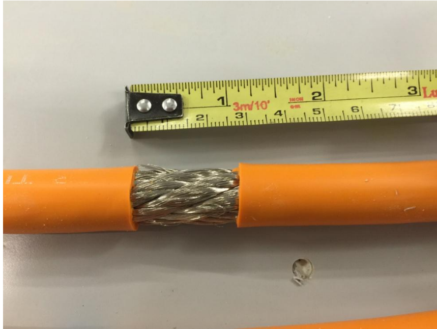
Image 3: 1 inch of duraelectric jacket removed for Autoshrink installation.
